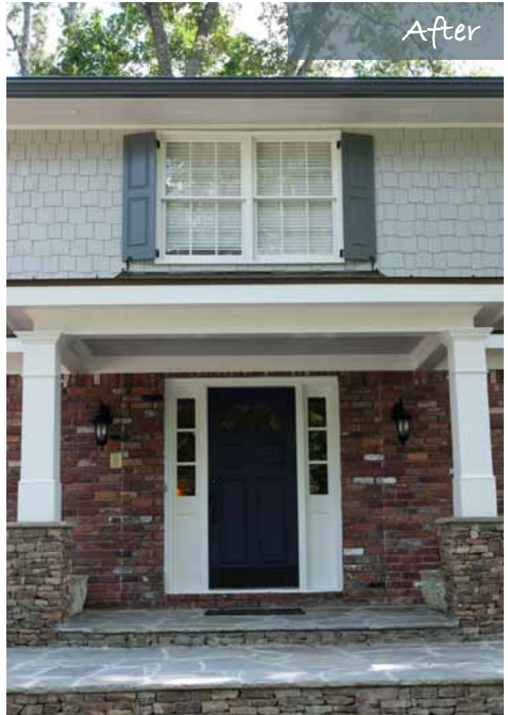
Addition of portico with curved metal hip bay top, bead board ceiling and PVC columns with stacked stone pedestals.
